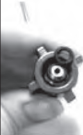
CO2 line to regulator
